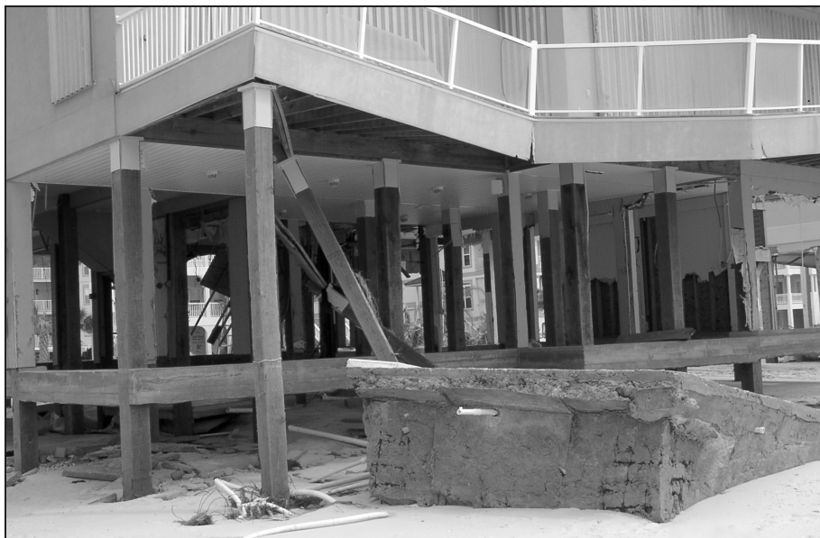
Figure 18. Movement of a spa likely caused failure of two piles supporting an elevated deck.
