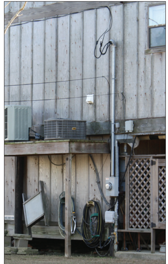
Figure 1. Electrical components installed below the lowest floor system are subject to increased flood damages and lengthy outage durations (St. Tammany Parish, LA)
