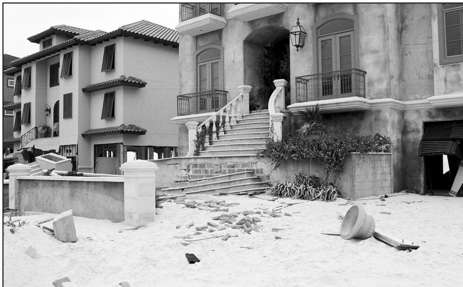
Figure 4. Non-compliant stairs
